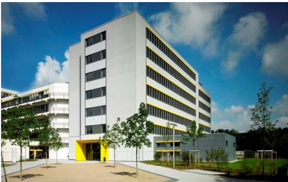
The building S07 at the Essen campus houses almost 100 modern chemistry laboratories.
