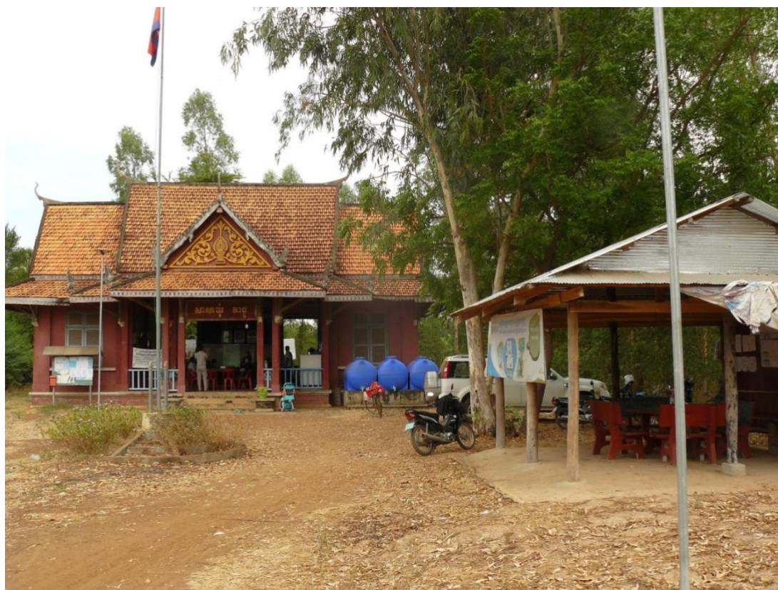
Fig. 5: Typical commune administration building, as constructed under an ADB programme in all six sample provinces.
