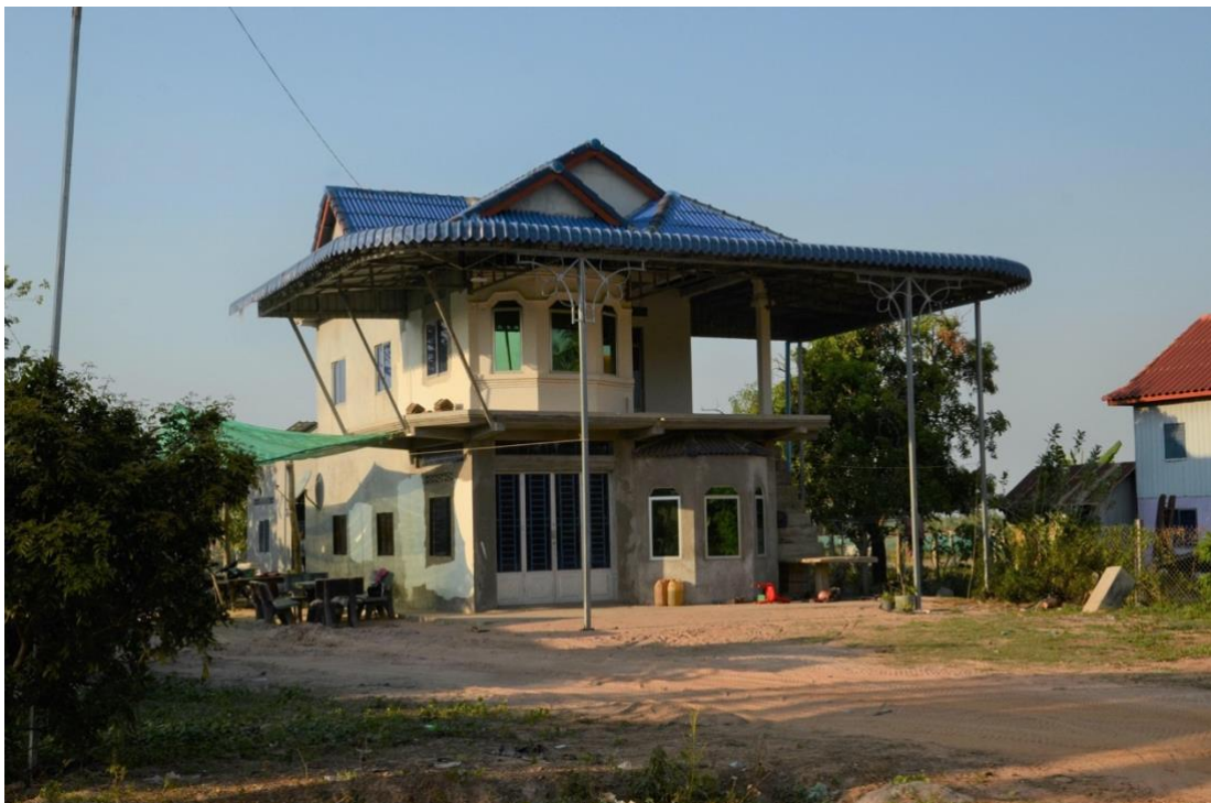
Fig. 12: The somewhat futuristic-looking new construction of a residential building, for which a long-term loan was taken out at more favourable conditions (10% instead of 18% interest rate).
