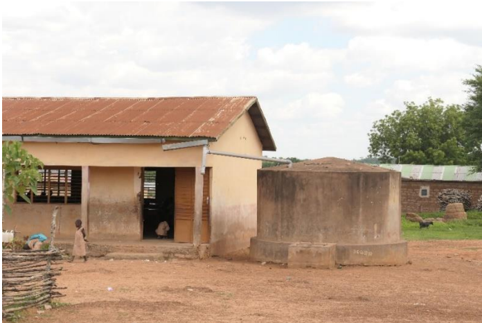
Fig. 31: Rainwater collection device with defective downpipe.
