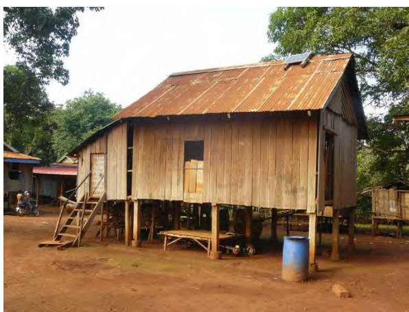
Pict. 2: Typical house made of wood, on poles because of the floods prevalent during the rainy season in the northern provinces of Cambodia
