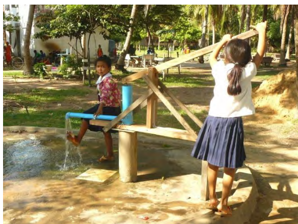
Pict. 3: The only water well of a primary school in the north of Kampong Thom, a simple manual pump with a maximum of 8 m lifting height
