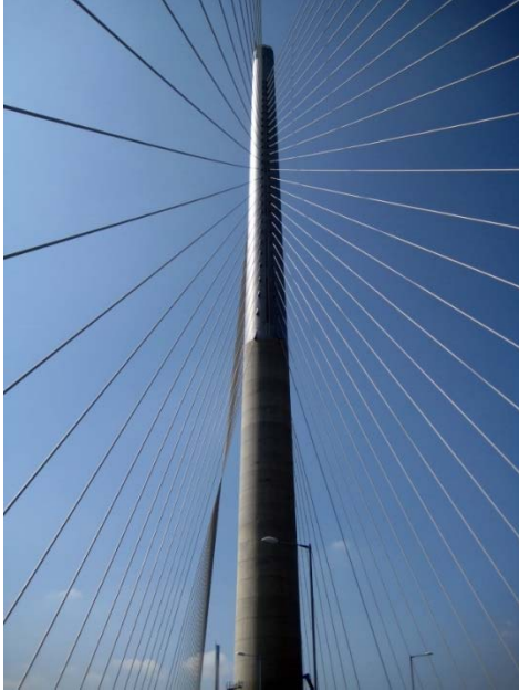
Figure 1.3 One of the two Stonecutters Bridge towers with the stay cables (Photo: Arup)
