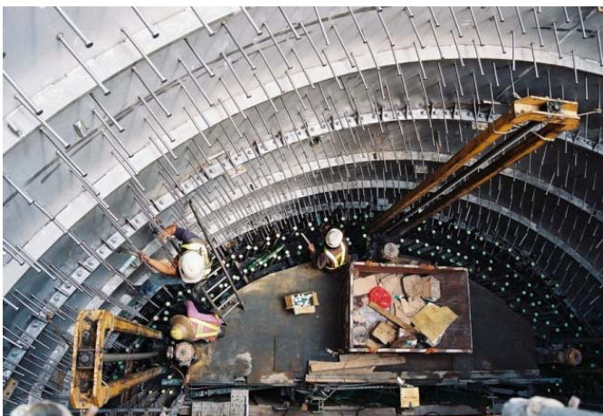
Figure 1.4 Shear connectors on the inside of a tower segment (Photo: Arup)
