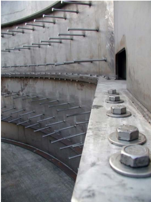
Figure 1.5 Edge flange connection (Photo: Arup)
