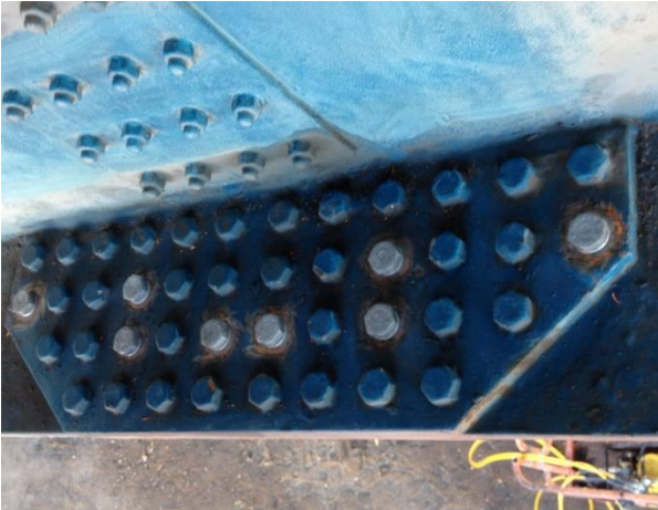
Figure 35 - One side of the connection after installation of the new bolts
