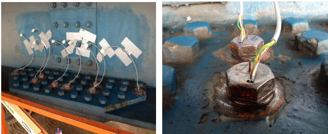
Figure 33 –Bolts with their installed strain gauges
