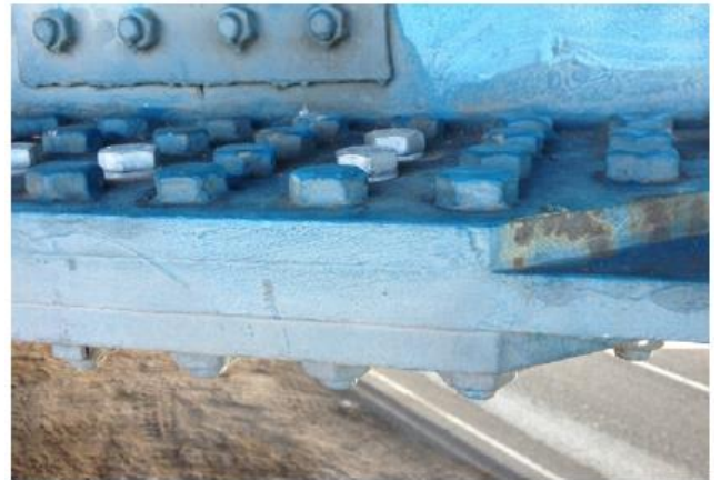
Detail of the joint the method was tested on. Measurements were carried out on M24, HV10.9 bolts with a total clamp length (washers + steel plates: 4+24+32+24+4 ) of 88 mm.
