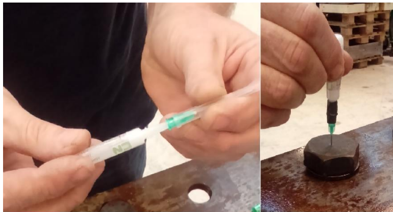
Figure 24 – Injection of CN adhesive using a syringe into pre-drilled hole
