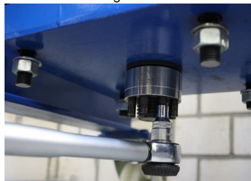
(e) increasing the load level by using Superbolt
