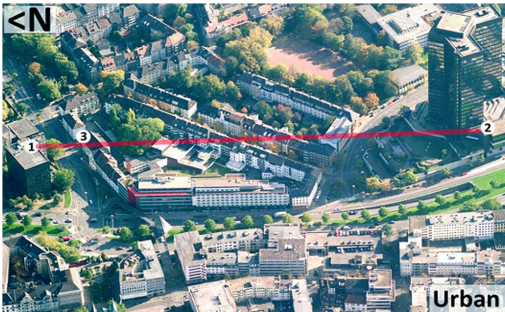
Fig. 1: Open-path CO 2 measurement (total length 704 m) in the city centre of Essen, Germany. 1: Sending/receiving unit; 2: Retro reflector; 3: open path of 704 m length at 34 m a.g.l.
