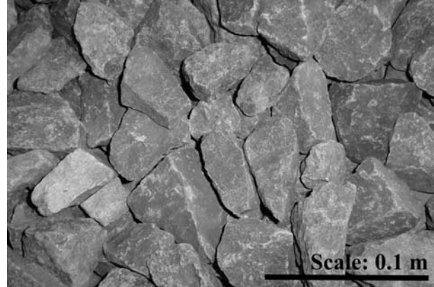
Fig. 1. Ballast surface at the study site in Osnabrück
